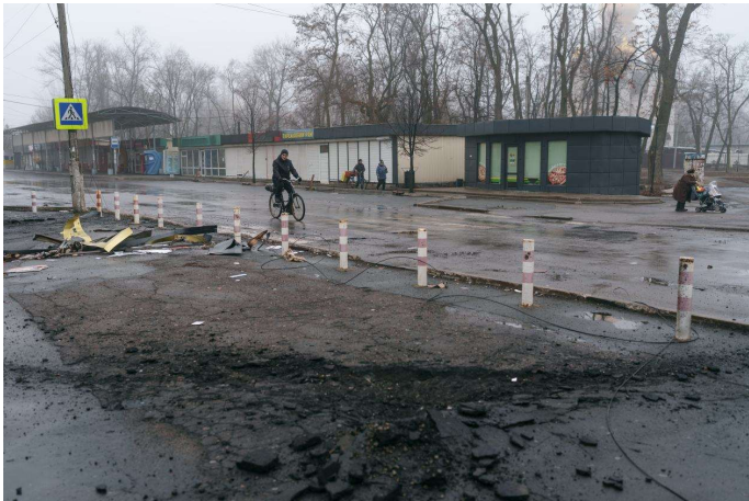
Destruction in the Ukrainian front-line town of Pokrovsk. Photo: Serhii Korovayny for WSJ
