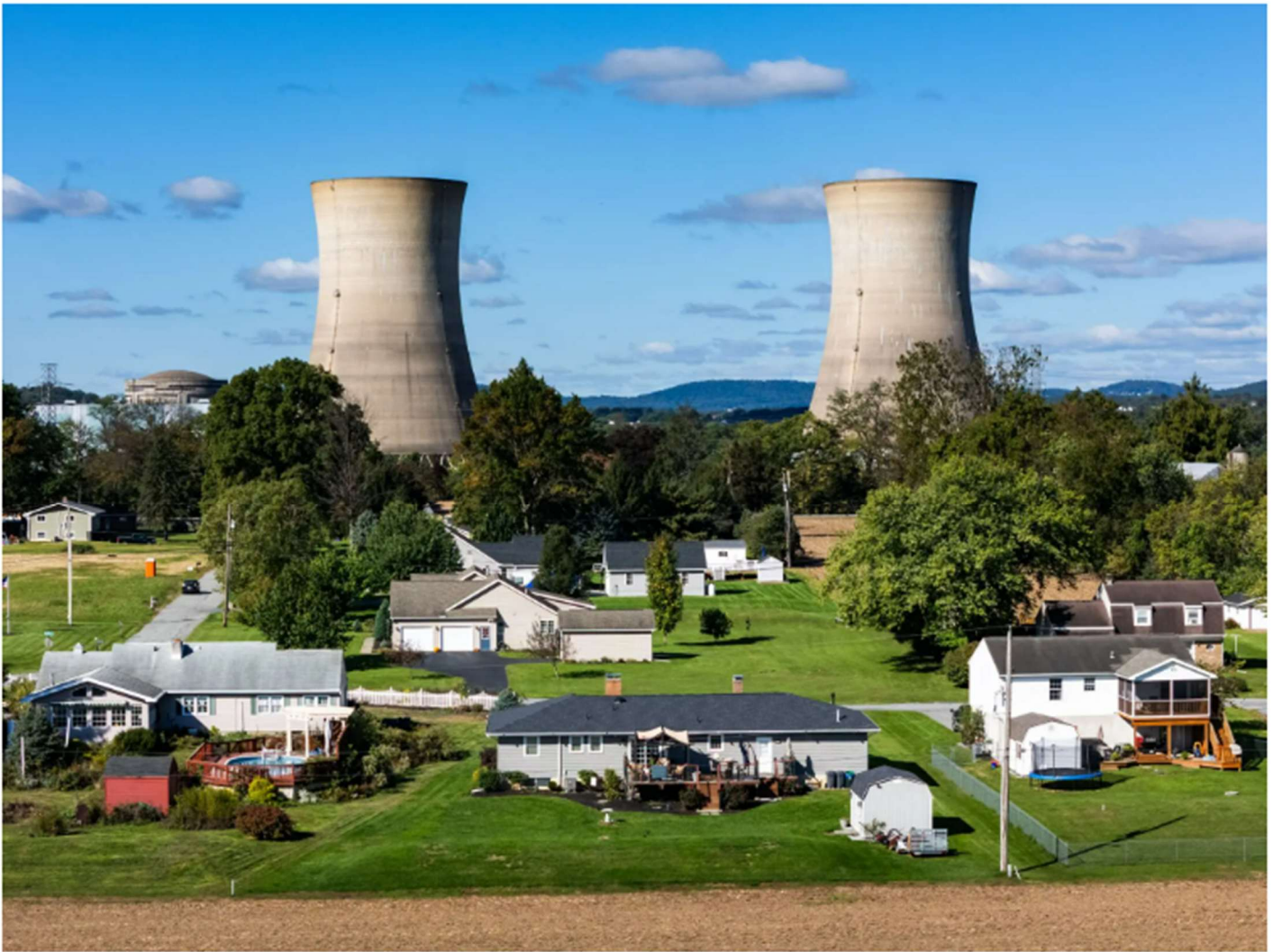
Cooling towers at the shuttered Three Mile Island nuclear power plant near Middletown, Pa., last month. One reactor will be brought back online in 2028. Jim Lo Scalzo/EPA, via Shutterstock
