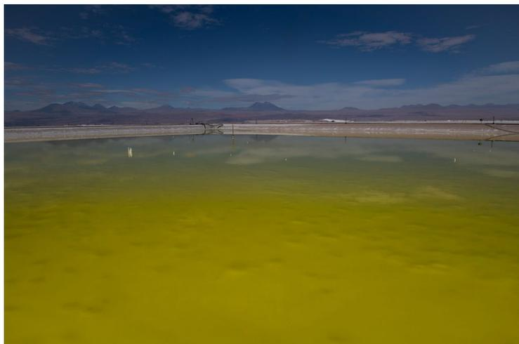
*A brine reservoir, a step in the lithium-extraction process.*
